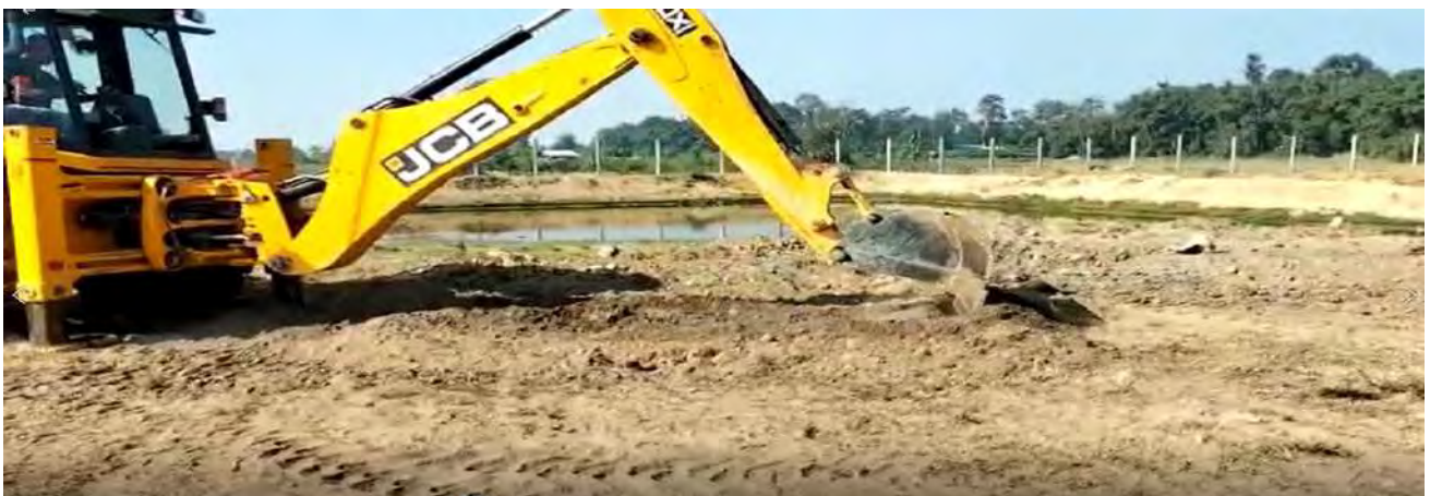
Tilling and mixing of microbes in soil by JCB machine inside plinth fenced area at BGN-5, Baghjan.
