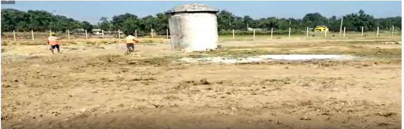
First phase microbes application inside plinth fenced area at BGN-5, Baghjan.
